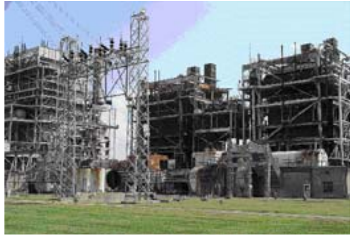
This former industrial facility, located on the southwest portion of the 574-acre tract, was retired in 2002. Nine recognized environmental conditions were identified in the Phase I Environmental Assessment.
