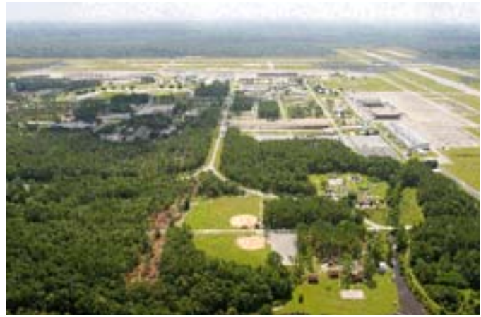
Cornerstone conducted a Megasite study to identify larger sites for major projects and has assisted in moving them to a shovel-ready status. Cecil Commerce Center on the Westside of Jacksonville is one of those sites ready for development.
