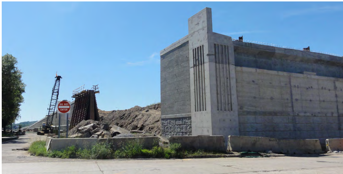
Construction of decorative bridge abutment in Riverview
