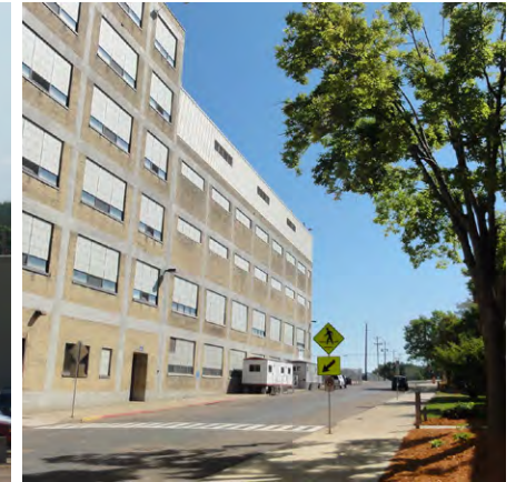
Former 3M Warehouse
