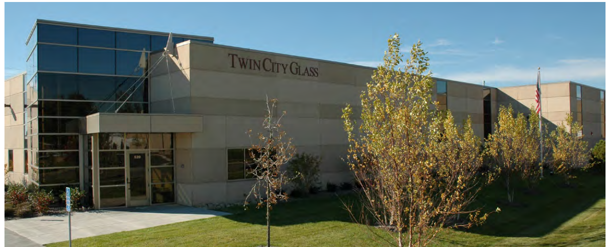
Twin City Glass Contractors, Great Northern Business Center
