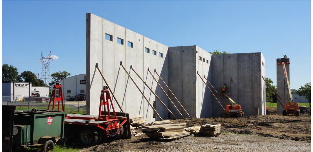
New industrial development under construction at Chatsworth
