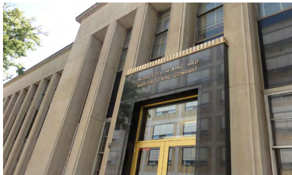
Former 3M Administration Building at Beacon Bluff
